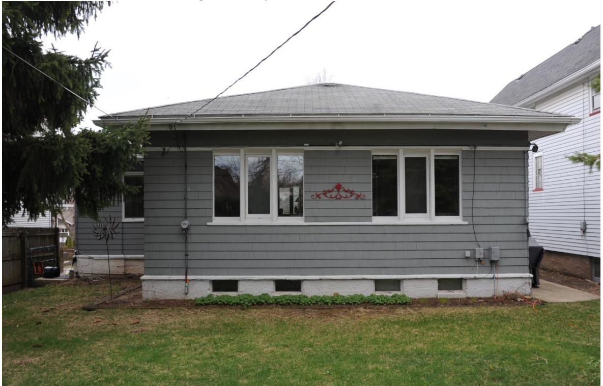
2106 Newton, rear View, facing South - April 22, 2015
