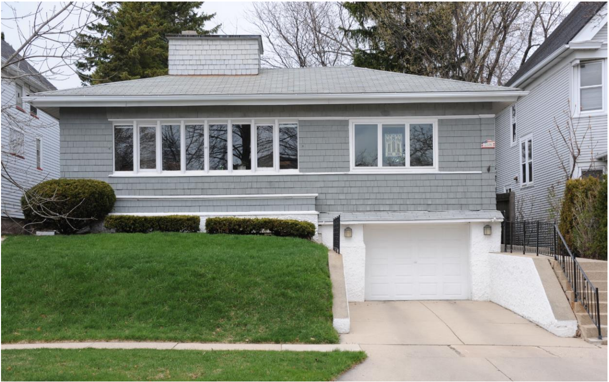
2106 Newton, Street View, facing North - April 22, 2015
